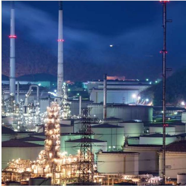
Industrial application: Refinery
