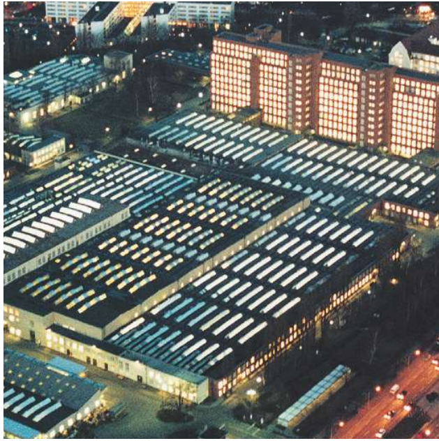
Switchgear Factory in Berlin, Germany
