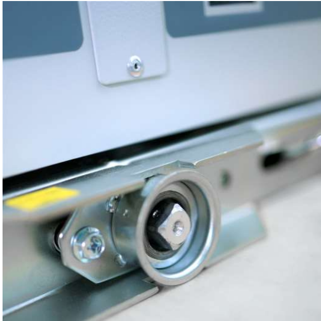
Racking interface of Compact CFC withdrawable module
